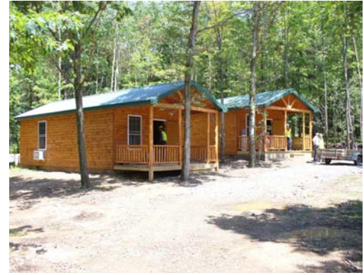
The new cabins - Three days before campers arrived we were given occupancy permits for the final cabins.
